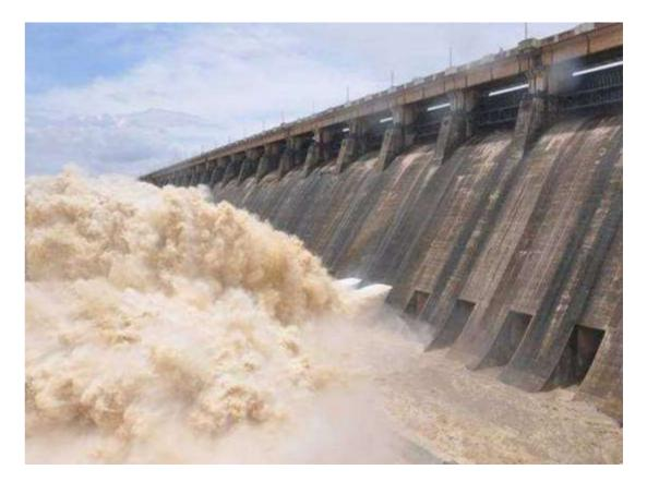
Energy dissipators are devices designed to protect downstream areas from erosion by reducing the velocity of flow to acceptable limits.
